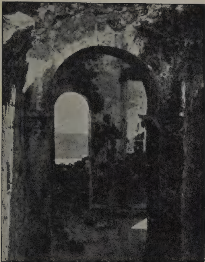
FIG. 304.—Sivri Hissar, N. aisle looking E., showing vault.
